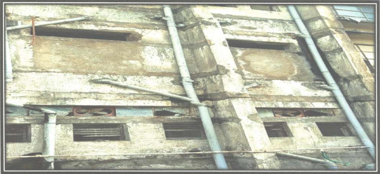
Maintenance of water system
