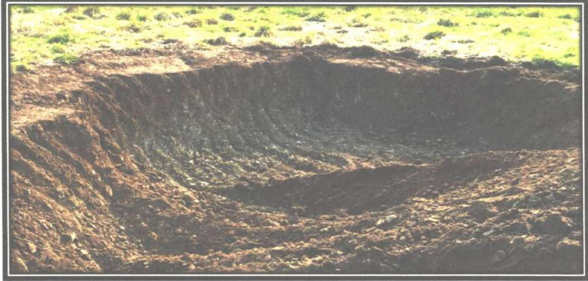
Rainwater Drainage Facility
